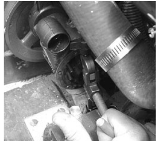
Removing the old impeller with the Jabsco puller.
