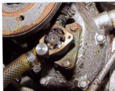
Old cover gone, new slide-on bolts in place
