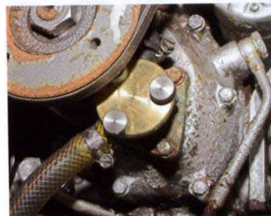
Speedseal in place, ready for emergencies
